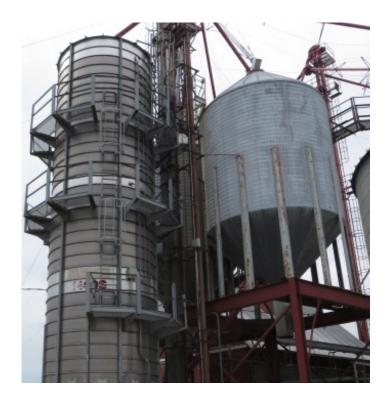
In order to reduce the risk of fire, grain material should be regularly cleaned from the inside and outside of grain dryers. The air intake screens should be kept clean and in good condition to prevent combustible material from being drawn into the dryer.
